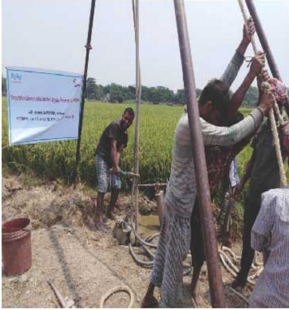
Figure-5: Runrig Soil Boring Works
